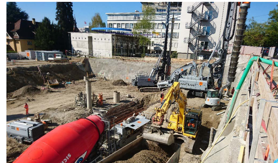
Baugrube Stand April 2017 / smt
