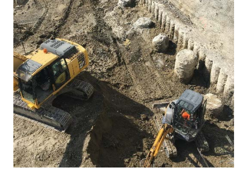
Baugrube Stand April 2017 / smt
