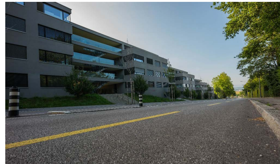
Deckbelags AC MR 8
